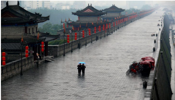
City Wall/ Cycling on the wall
